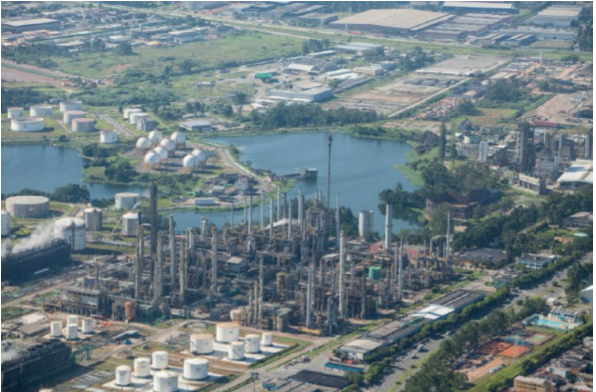
The ABC Petrochemical Complex in São Paulo is powered by a cogeneration plant that is fueled by residual process gas with a very high content of hydrogen.
